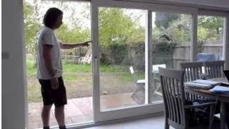
Lift and slide doors have the benefit of sealing like a hinge door, they have a low threshold. They are suitable for wheelchairs.
